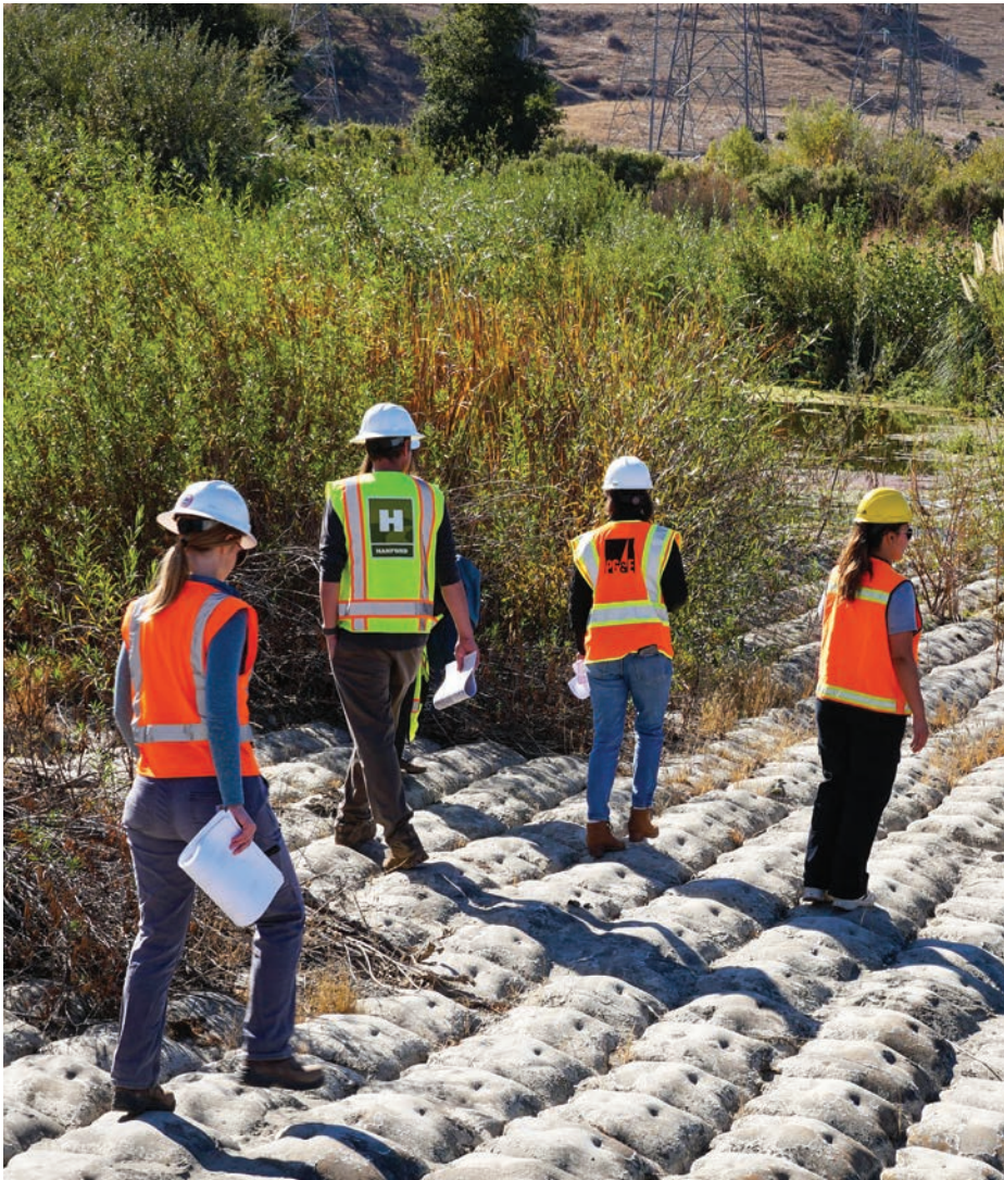
Officials inspect the PG&E gas pipeline protective apron over Alameda Creek near Sunol. Photo by California Trout
