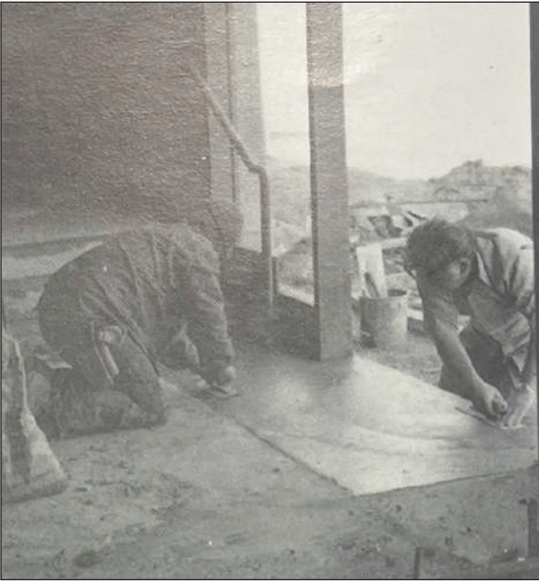
Students would greet the contractors putting on finishing touches. Courtesy of Sherry Wright
