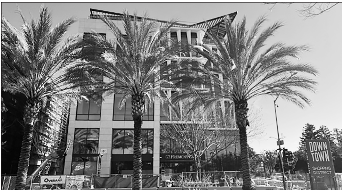
The new Fremont Bank Building features smart glass that can switch between transparent and opaque. Photo source: City of Fremont
