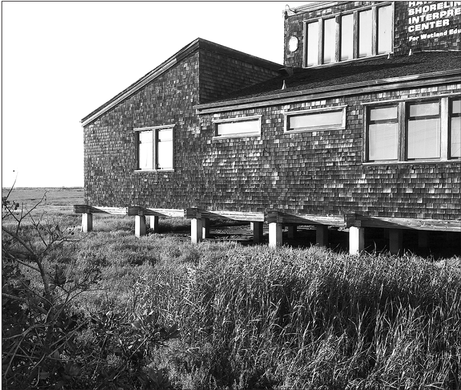
Hayward Shoreline Interpretive Center at high tide 1/04/2024. Photo By Jack Alcorn
