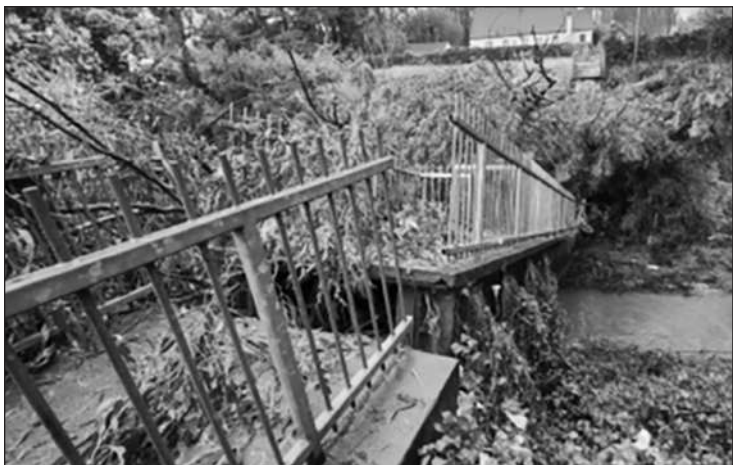
Haas Ave Pedestrian Bridge
