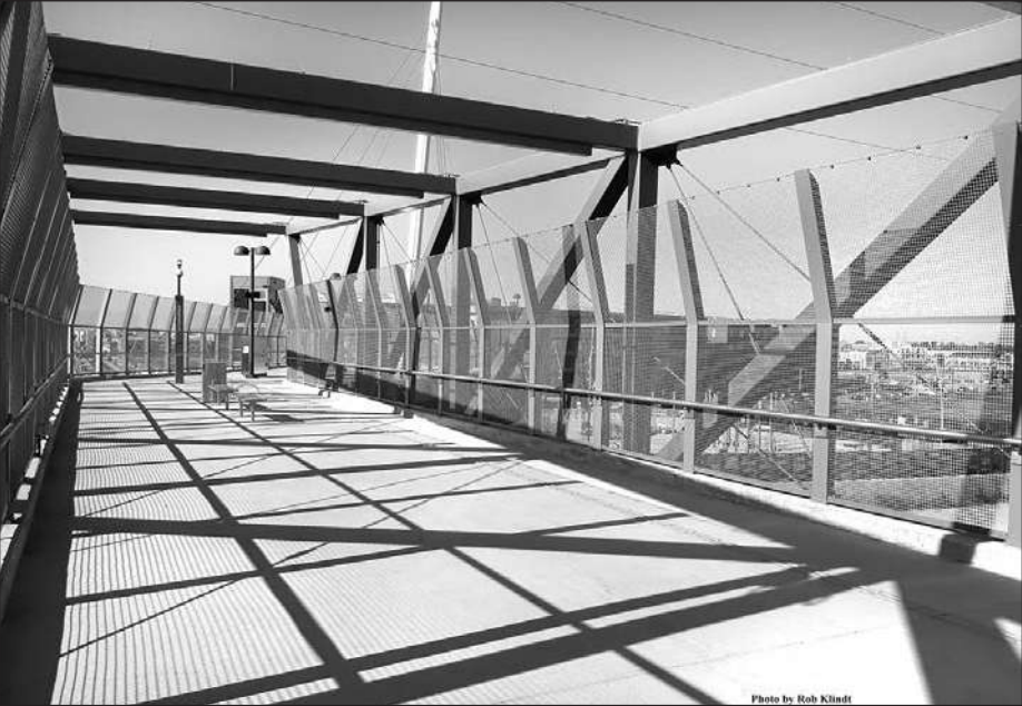
The bridge takes pedestrians over five railroad tracks.
