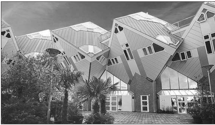
The homes of the future will be built to use a lot less energy and withstand harsher, more extreme weather events thanks to global warming. Credit: Karin S, Pexels.com.
