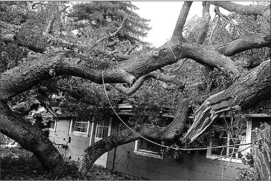
A Castro Valley home was damaged when large tree fell onto it. Credit: Alameda County Sheriff’s Office/Facebook
