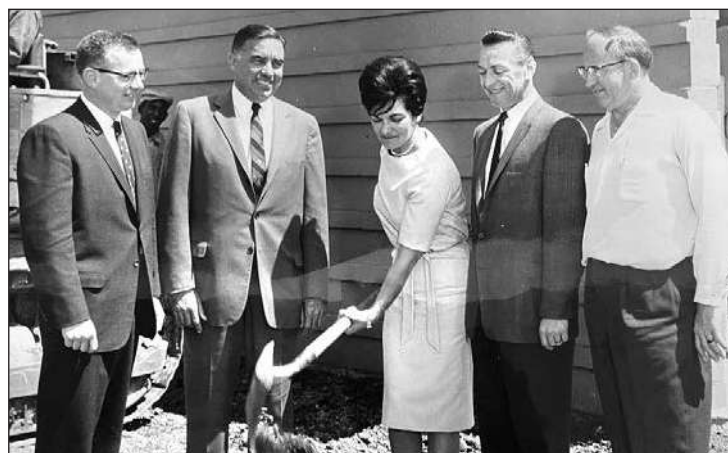
The Hillmans break ground to add 12 lanes to the bowling center in 1963
