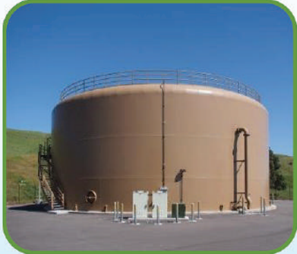
Appian Tank, Union City Retrofitted for earthquakes
