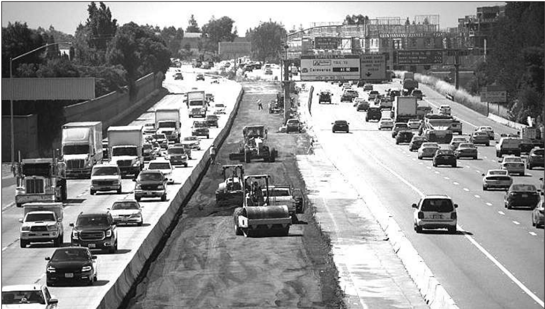
Northbound I-680 Express Lane construction in Fremont
