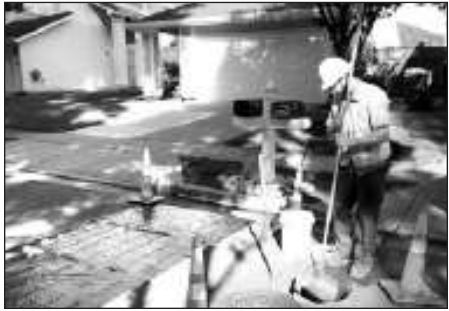
USD Collection System worker Walker Rollins retrieves wipes from USD's sewer main for the CASA wipes study. PHOTO: Jose Rodrigues Jr.
