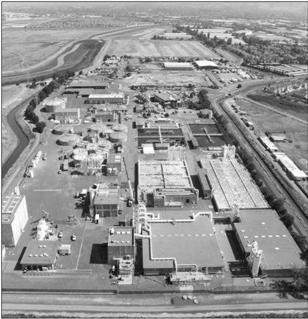
USD's Treatment Plant today
