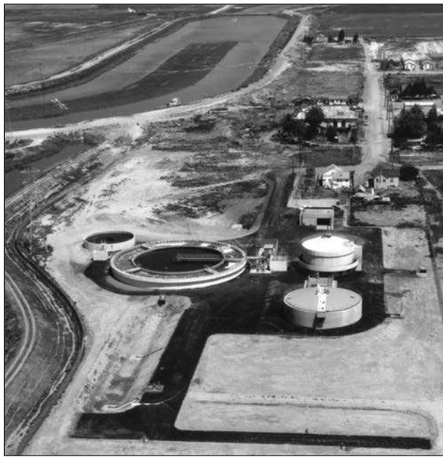
USD's Treatment Plant 1964
