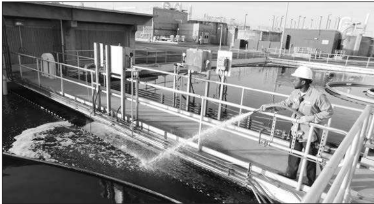
Lee cleans algae off a weir in a secondary clarifier
