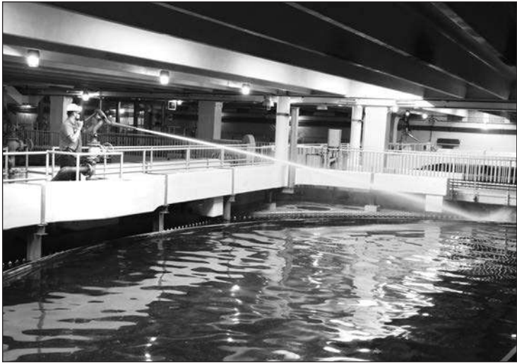
Fulkerson uses a high-pressure water nozzle to clean debris in a primary clarifier
