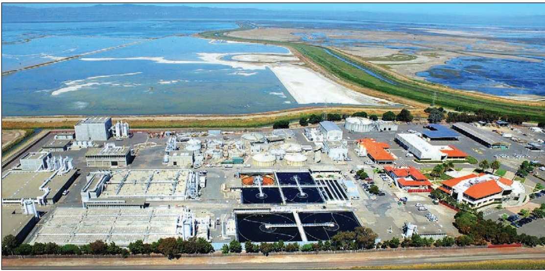
An aerial view of the Alvarado Treatment Plant at the Union Sanitary District Headquarters. Photo courtesy of Michelle Powell.
