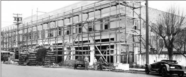
The addition that turned the “Eggert Building” into the “Green Shutter Hotel” under construction in 1926. This view is from Main Street looking north-east
