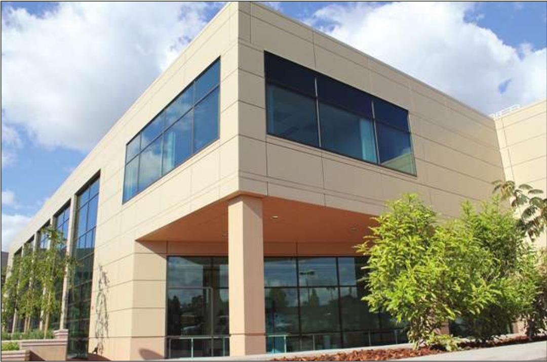
Construction of the Central Utility Plant, which opened in 2011, is a key component of the Hospital’s long-term facilities master plan. Voter-approved Measure FF bonds financed the construction of the plant, along with other facility improvements to help Washington Hospital meet earthquake safety standards by 2030. Refinancing of the general obligation bonds is saving district taxpayers $5.84 million over the remaining life of the bonds.
