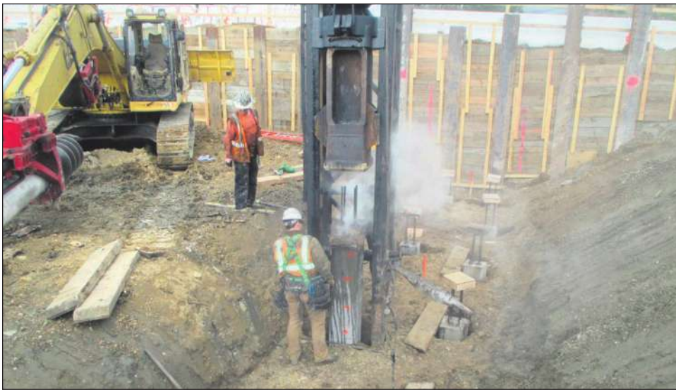
Pile driving at east side abutment
