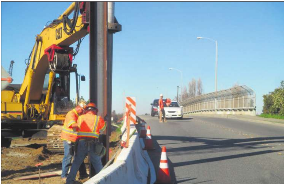
Drilling for temporary shoring at east side abutment
