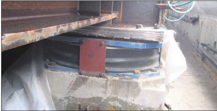
72 giant base isolators (shock absorbers) and 34 horizontal pistons called dampers, cushion the structure to absorb and reduce movement during an earthquake
