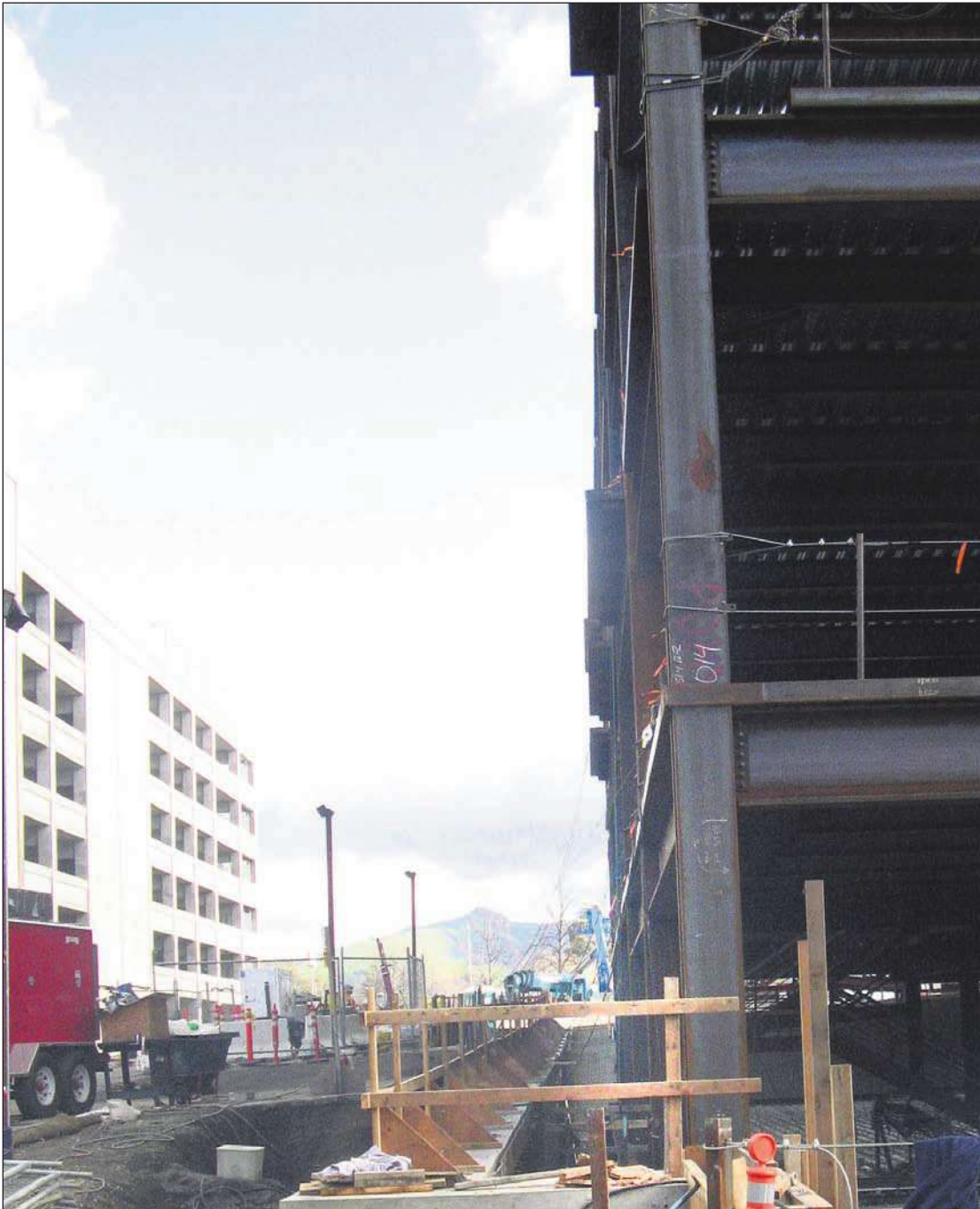
A three foot moat surrounds the building to allow horizontal movement and protects not only the structure but also connections with adjacent facilities.
