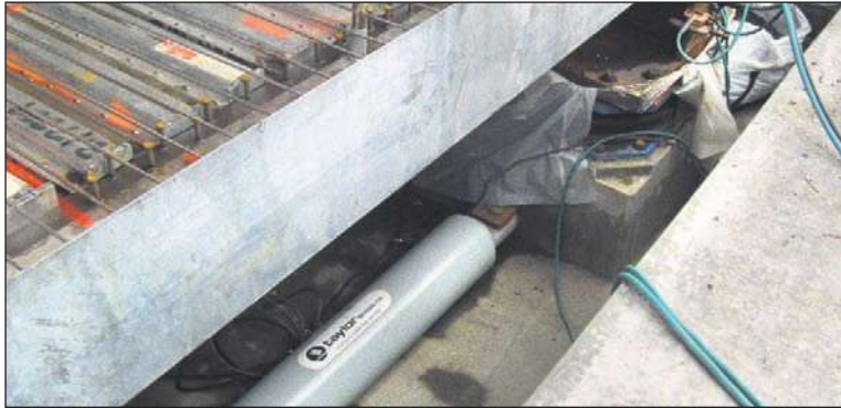
72 giant base isolators (shock absorbers) and 34 horizontal pistons called dampers, cushion the structure to absorb and reduce movement during an earthquake
