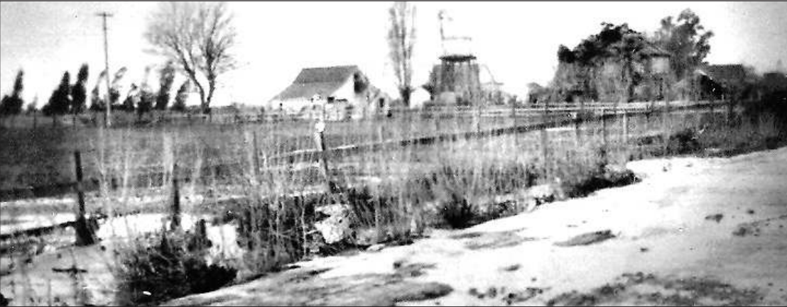
Beard ranch with flood on Alvarado Road 1996
