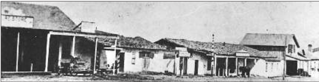
Mission San Jose Vallejo Street west side 1868
