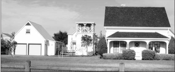
Hiram Davis House
