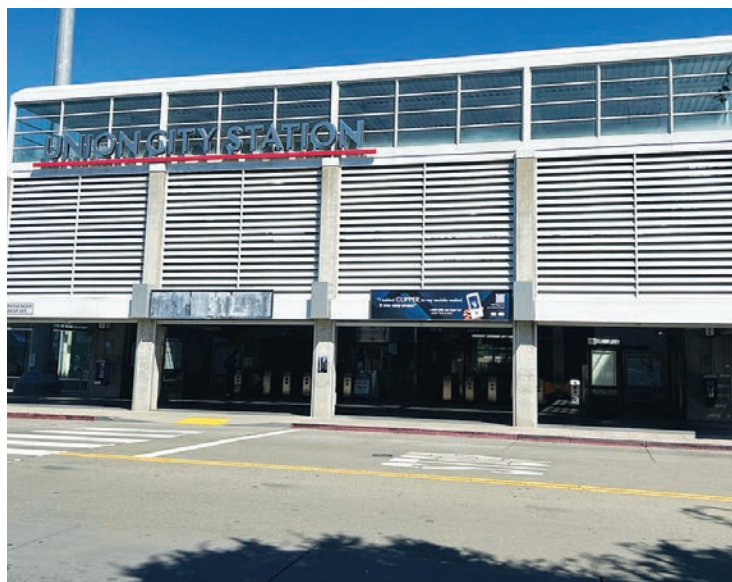
Union City officials held a meeting to reveal BART construction plans to the public. Photo by April Ramos
