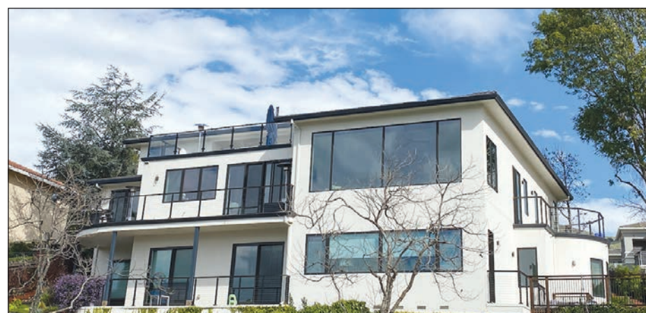
Large windows provide an impressive view from Vineyard Avenue
