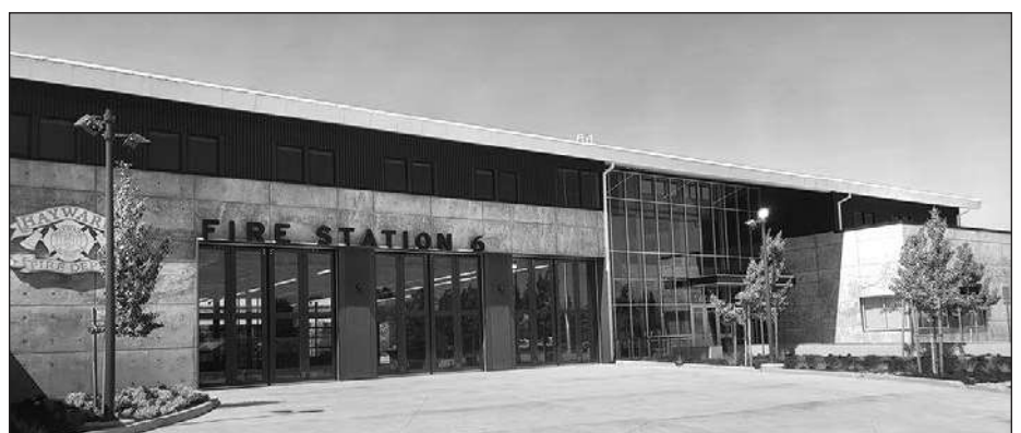
New Hayward Fire Station No. 6 and Training Center, Photo by Monika Lee
