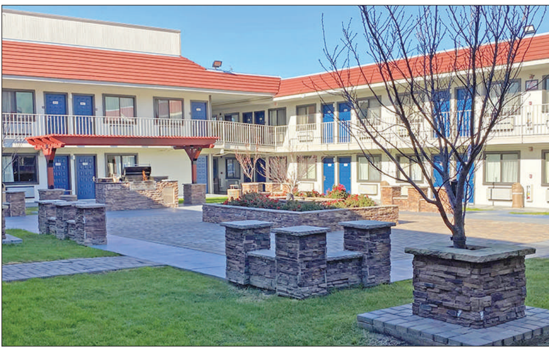
A Motel 6 in Fremont will be converted into permanent supportive housing Photo Credit: City of Fremont
