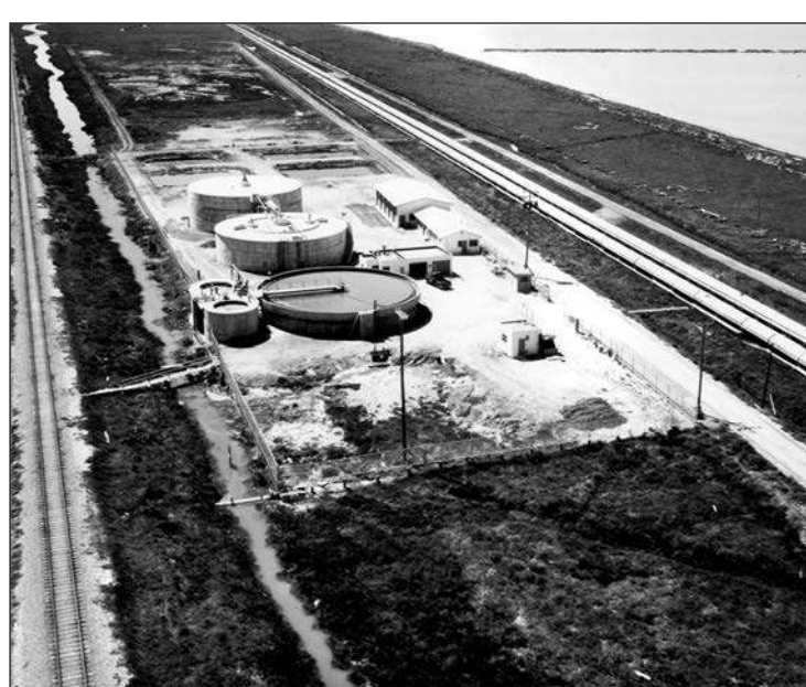
Newark treatment plant – late 1950s – early 1960’s
