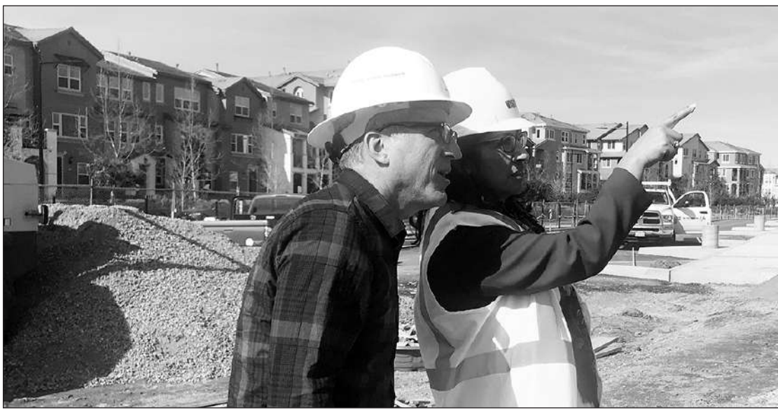
Director of Facilities Modernization Joe Flatley and Assistant Superintendent of Learning and Development Norma Rodriguez look out at the school construction site.
