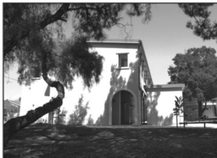
Board of Education approved the Notice of Completion for the new 12-classroom building at Warm Springs Elementary School
