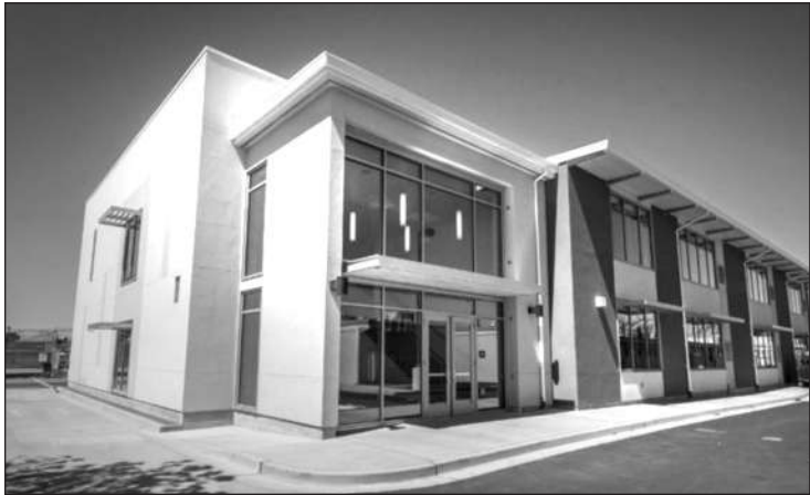
New Math/Science building at Irvington High
