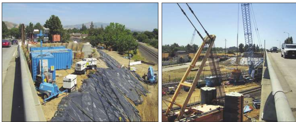
Cast in Drilled Hole (CIDH) pile installation is underway
