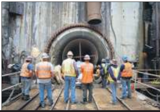
Bay Tunnel begins delivering Hetch Hetchy water
